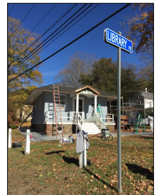
Library roof replacement and primed for paint
