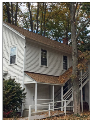
Museum's new roof
