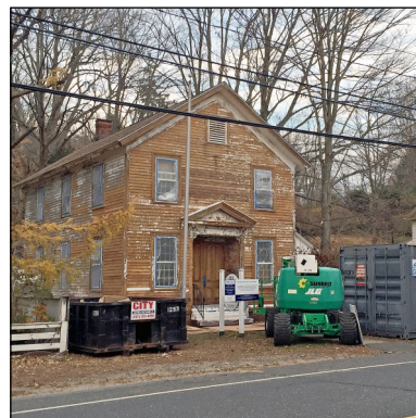
Museum stripped and ready for painting
